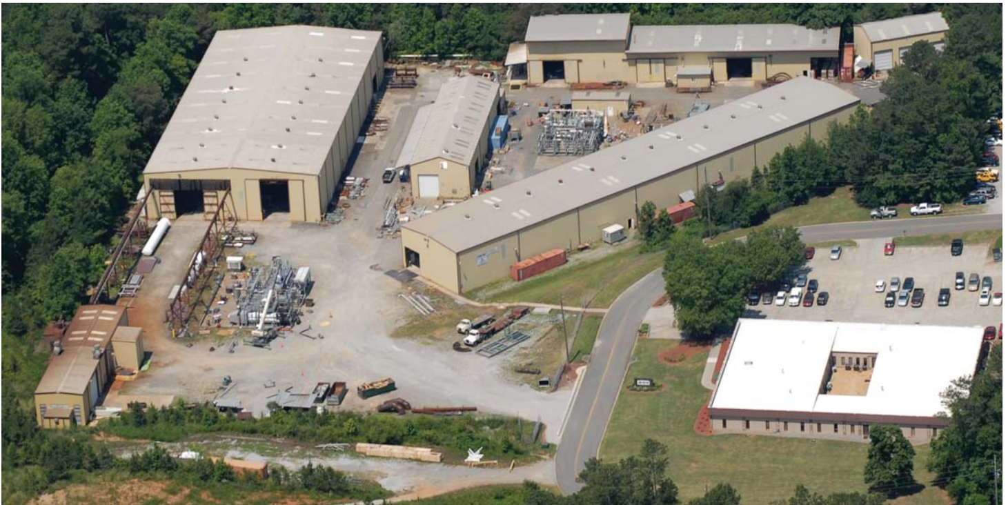
Hydro-Chem's fabrication facility and offices in Holly Springs, GA.
